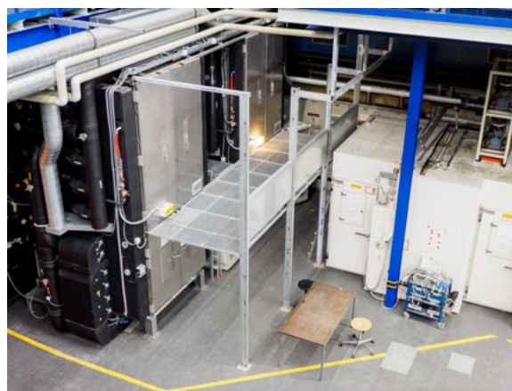
Figure 8.1: View of the hall where the sun simulators are located, in a redeployed building that used to be the home of a small nuclear reactor.
